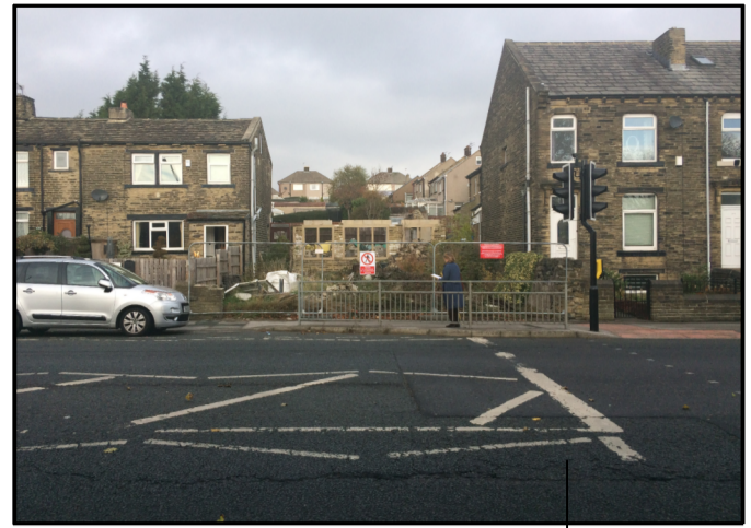
PHOTOGRAPH OF EXISTING STREET VIEW
